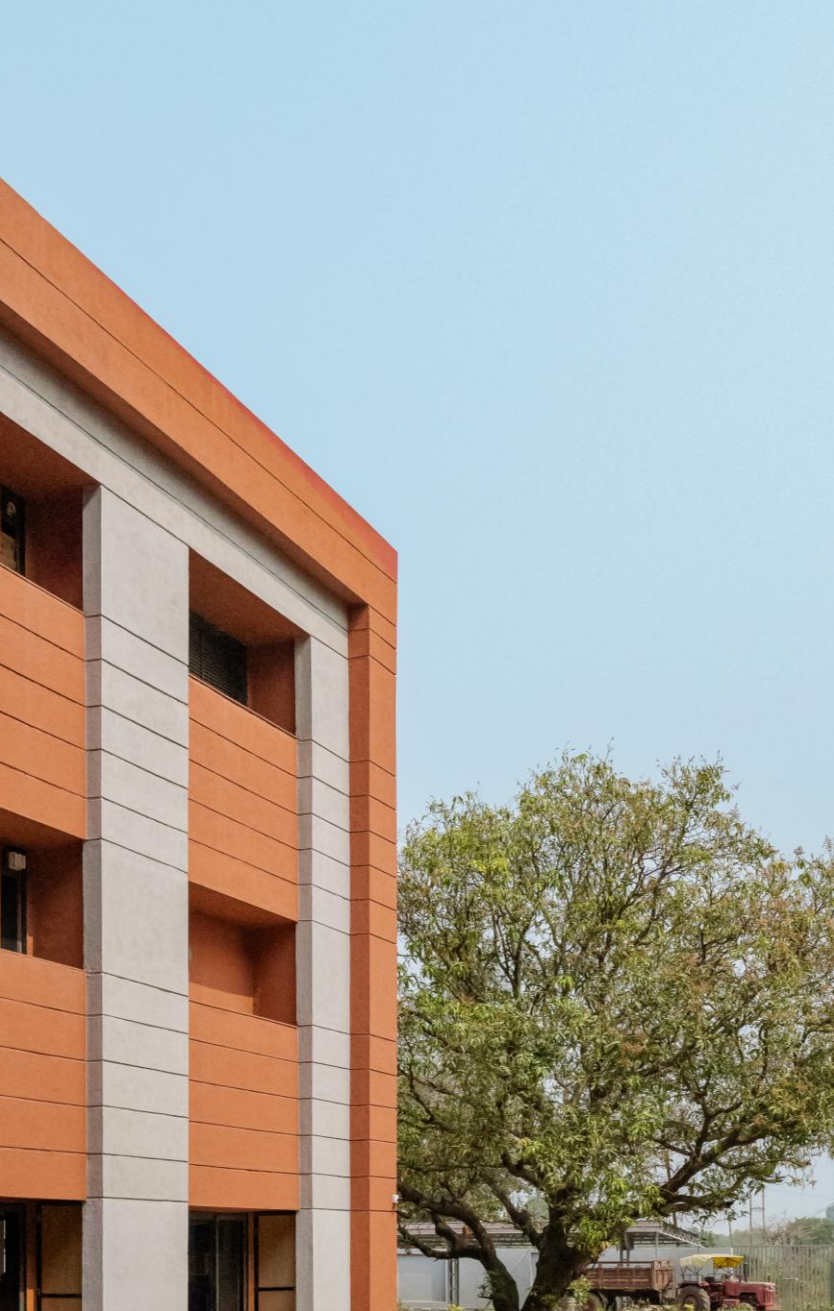
EXTERIOR DETAILS – DOUBLE SKIN FACADE & DEEP SEATED WINDOWS
