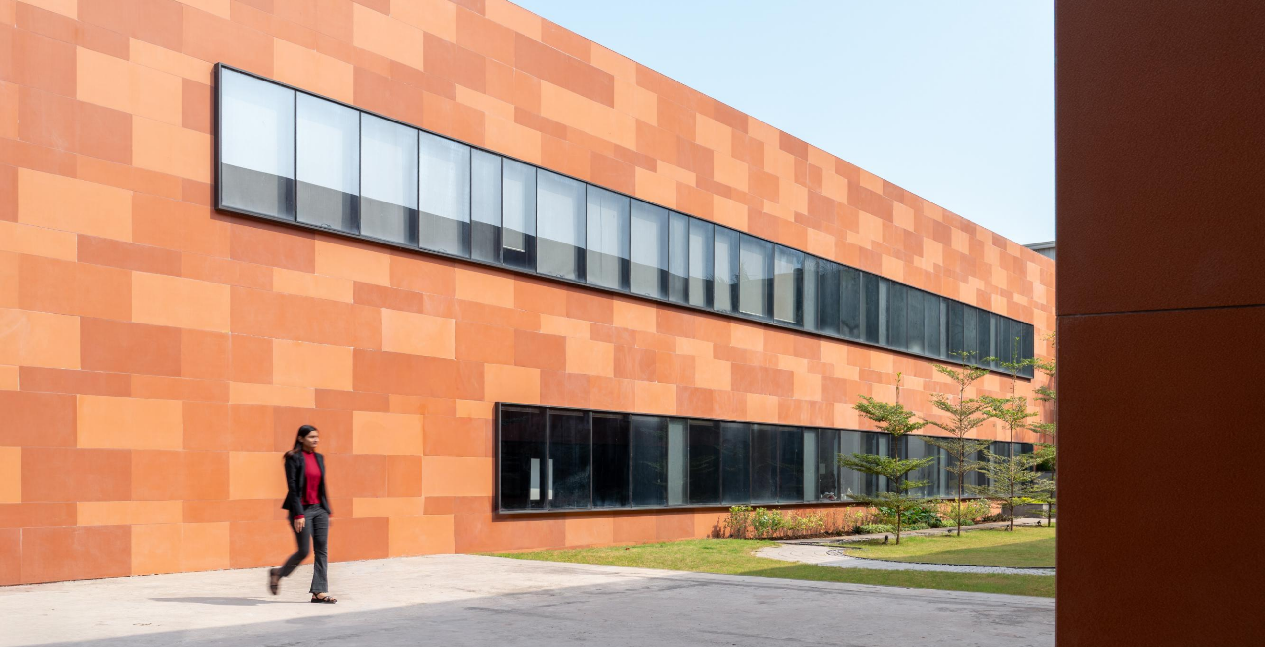
PASSAGE BETWEEN ADMIN BUILDING AND R&D BUILDING
