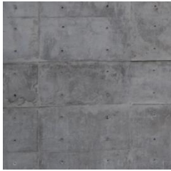
FORM FINISHED CONCRETE
